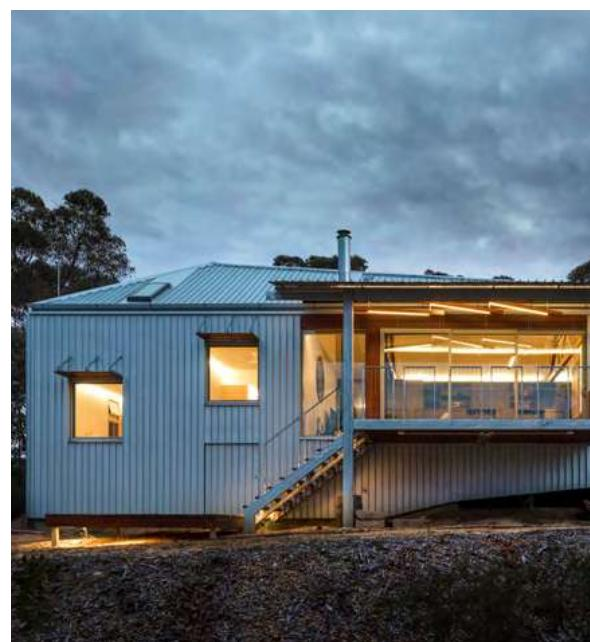
house, and all hardwood was repurposed as feature joinery, sunshades, privacy screens, decking and cladding. Finally, new materials, when needed, were selected to have the lowest embodied energy for their functional purpose. As such, all new internal framing, structure and linings are timber. Fibre cement sheeting is used in wet areas and behind the fireplace, and Zincalume cladding meets bushfire requirements.
